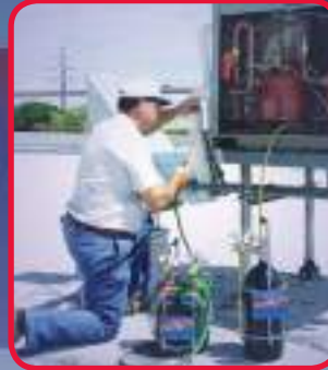
Purge and pressure test an A/C&R system
